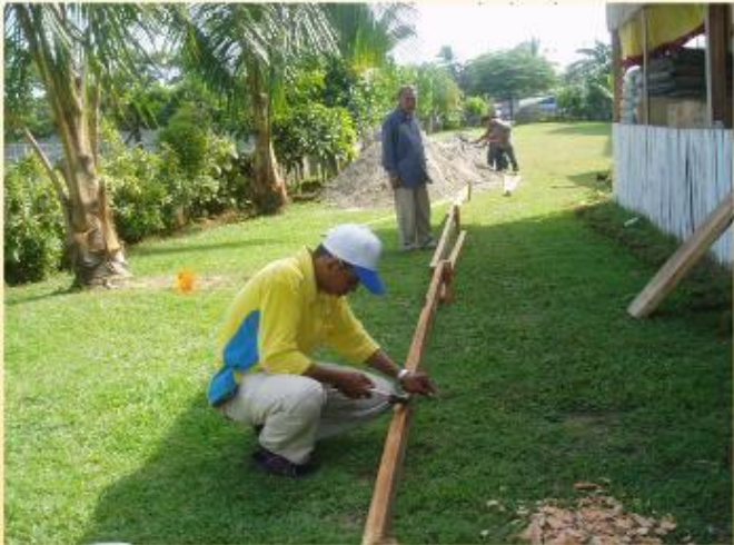
Below: Brother Jorge Prajeli of Barra church (in yellow shirt) is preparing the layout of the building
