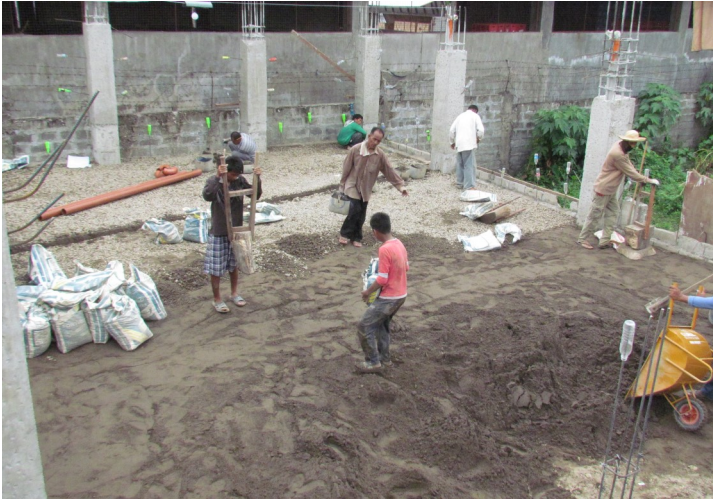
Ready for the sanctuary concrete floor
