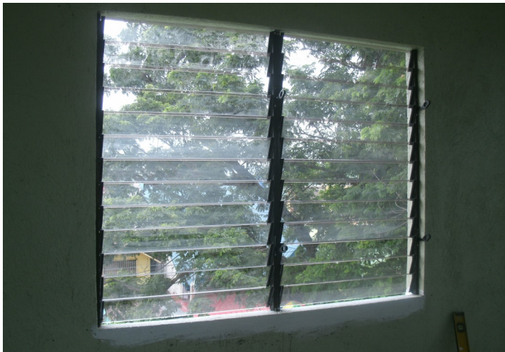
The finished interior walls on the second floor
