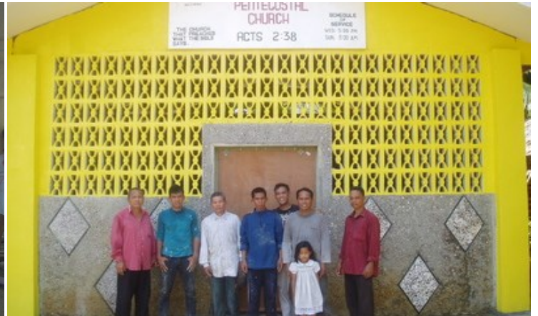
The Jimenez church was repaired and remodeled
