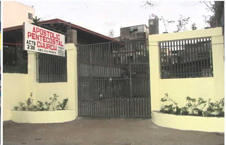
A new wall and gate for our new church property in Taguig City
